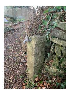
There may be a requirement to dig a trench to find the pipe and repair the leak or remove this standpipe altogether or cap off the pipe and locate a new tap in a better location.
